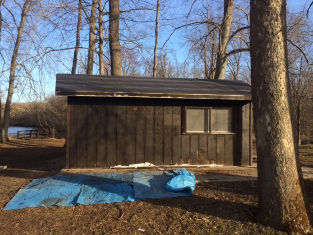
Boat Rental Building at Burchfield Park
