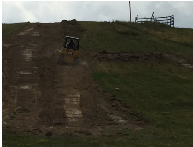
“Touching Up” rough areas on tubing hills and adjusting slope for arrival of Magic Carpet
