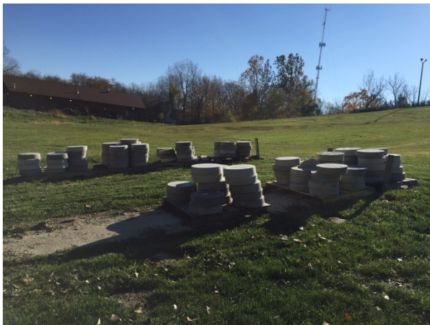
Concrete footings awaiting arrival of Magic Carpet snow tubing lift.
