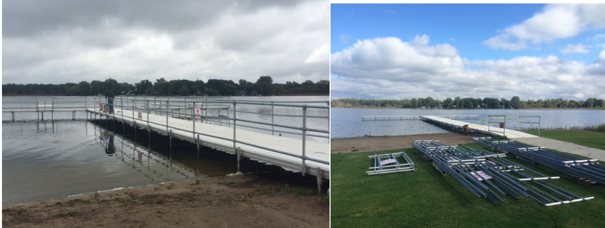
Removing dock railing for overall dock removal
