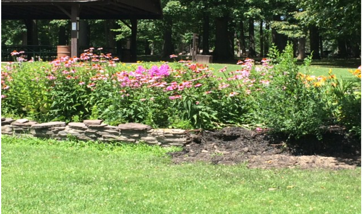
Replacing failed 10 year old retaining wall
