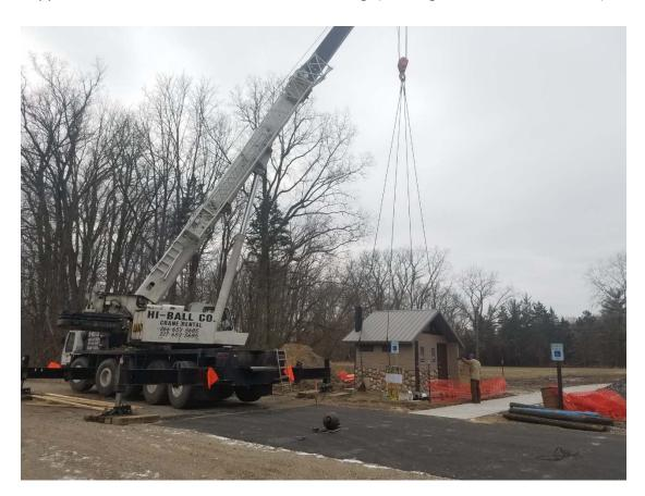
CXT restroom building being installed near Overlook shelter.
