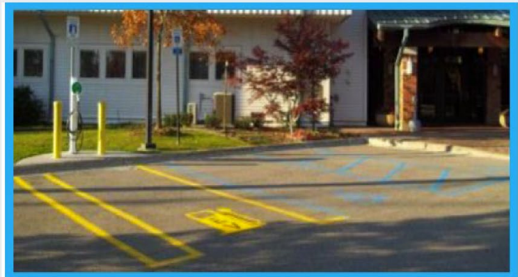
Figure 4.3 - Example of charging station next to ADA parking spot
