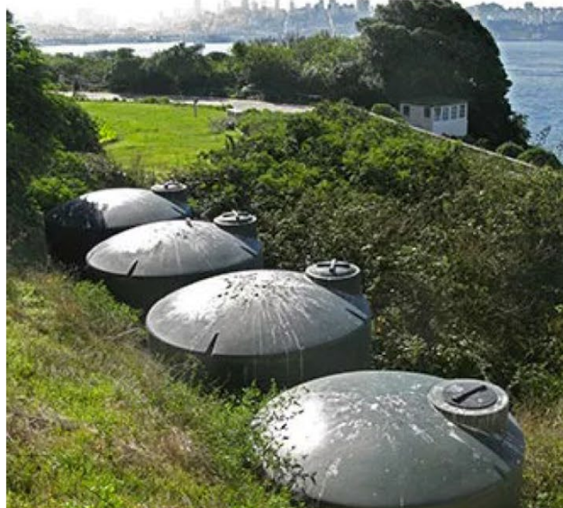
Akatraz Island uses a rainwater catchment system to capture water for landscaping the historic gardens on the island. Credit: NPS
