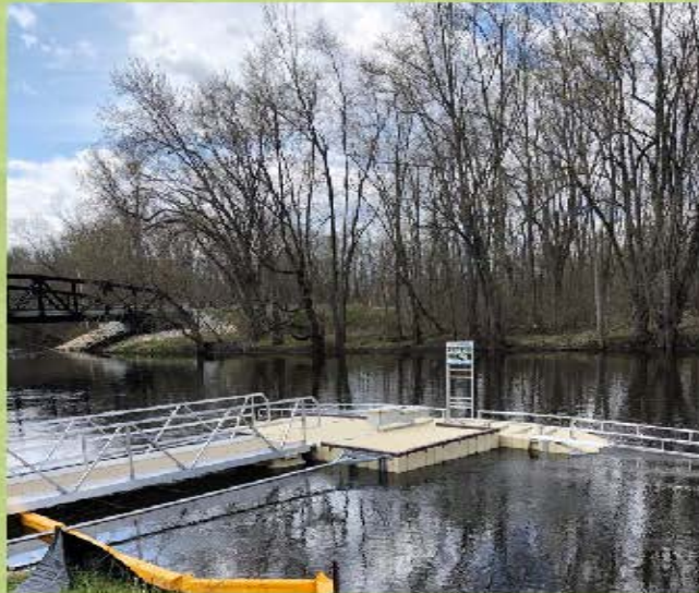
• New EZ Launch at McNamara Landing
