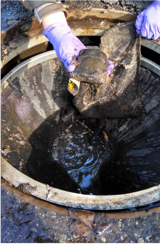
Figure 2: CB Insert Maintenance in District
