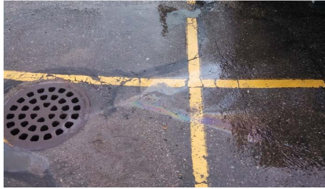
Figure 3: Oil Sheen in Parking Lot within the Drainage District
