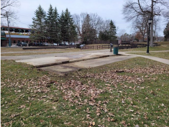
Trike storage and canopy removal
