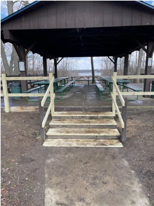
Lakeview steps and railing
