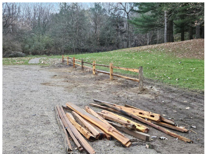
Pineknoll Split Rail Installation
