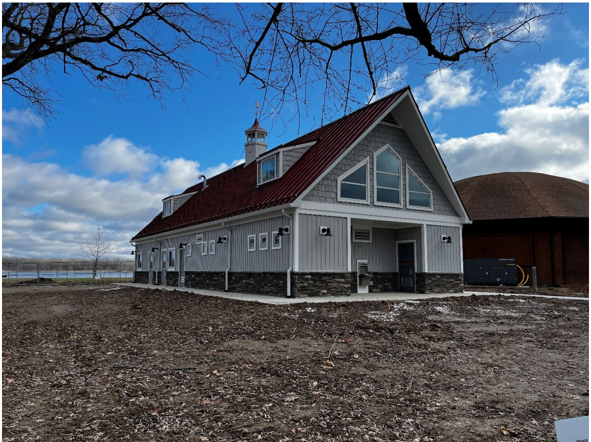
Lake Lansing South Concession and Bathroom Building looking like something from Parks and Recreation Magazine, a real showcase thanks to the MNRTF Funding and Land and Water Grants matched and made possible with the Trails and Parks Millage Funding
