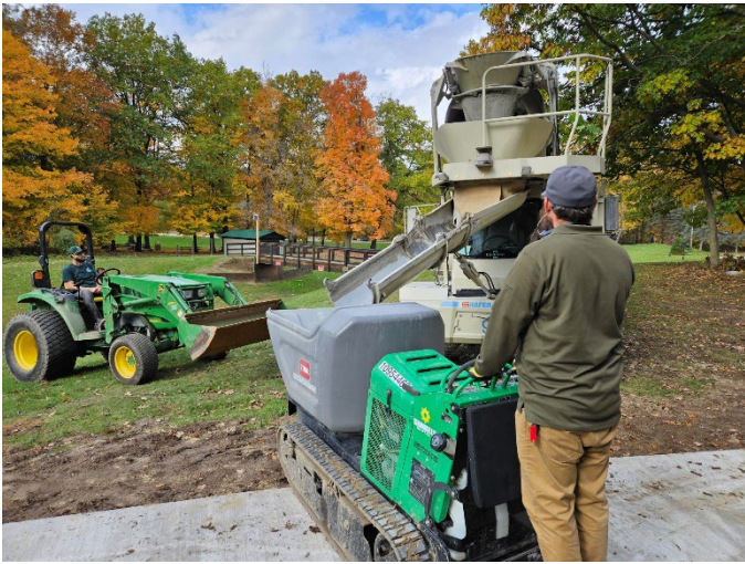
Power Buggy Moving Concrete
