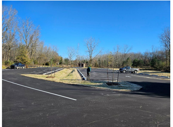
Completed McNamara Parking Improvements
