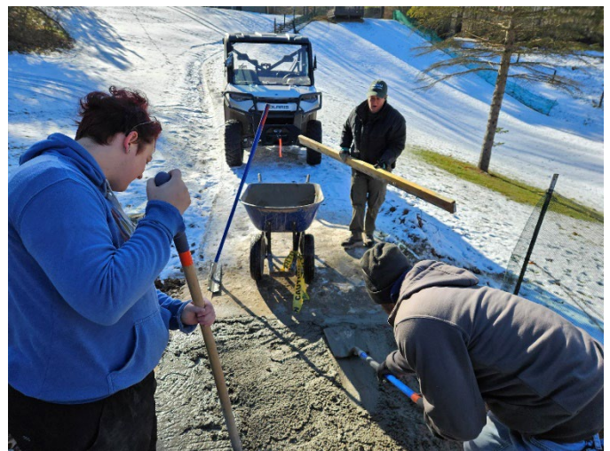
Sidewalk Completed Before Winter
