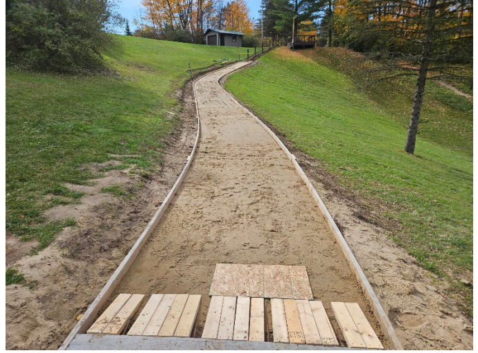
Forms in Place and Ready for Pour
