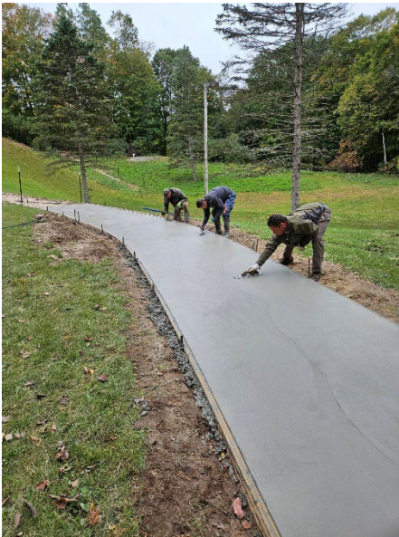
Finish Work on First Section
