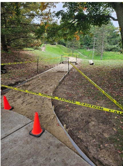
Concrete Forms for New Sidewalk
