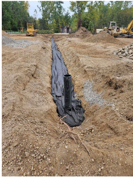
Parking Lot Runoff Retention Area
