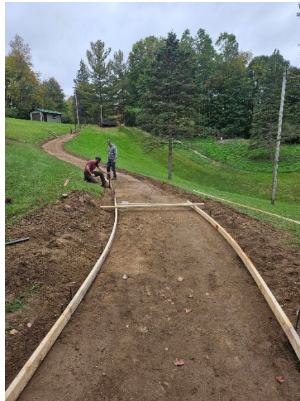
Prep Work on New Sidewalk
